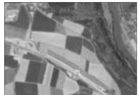
Photovoltaikpark Altfeld II
